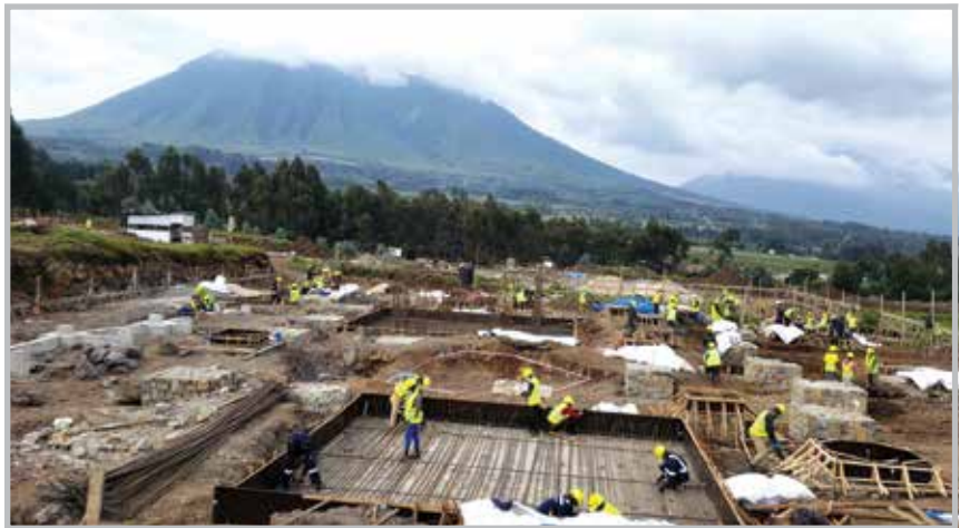
Above: Research Center. Settings for steel columns, stone masonry, drainage and other basic substructures are moving ahead quickly. This is where our science labs and research offices will be located.
