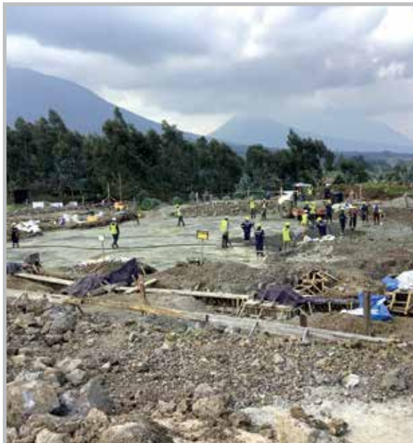
Above: Research Center. Settings for steel columns, stone masonry, drainage and other basic substructures are moving ahead quickly. This is where our science labs and research offices will be located.
